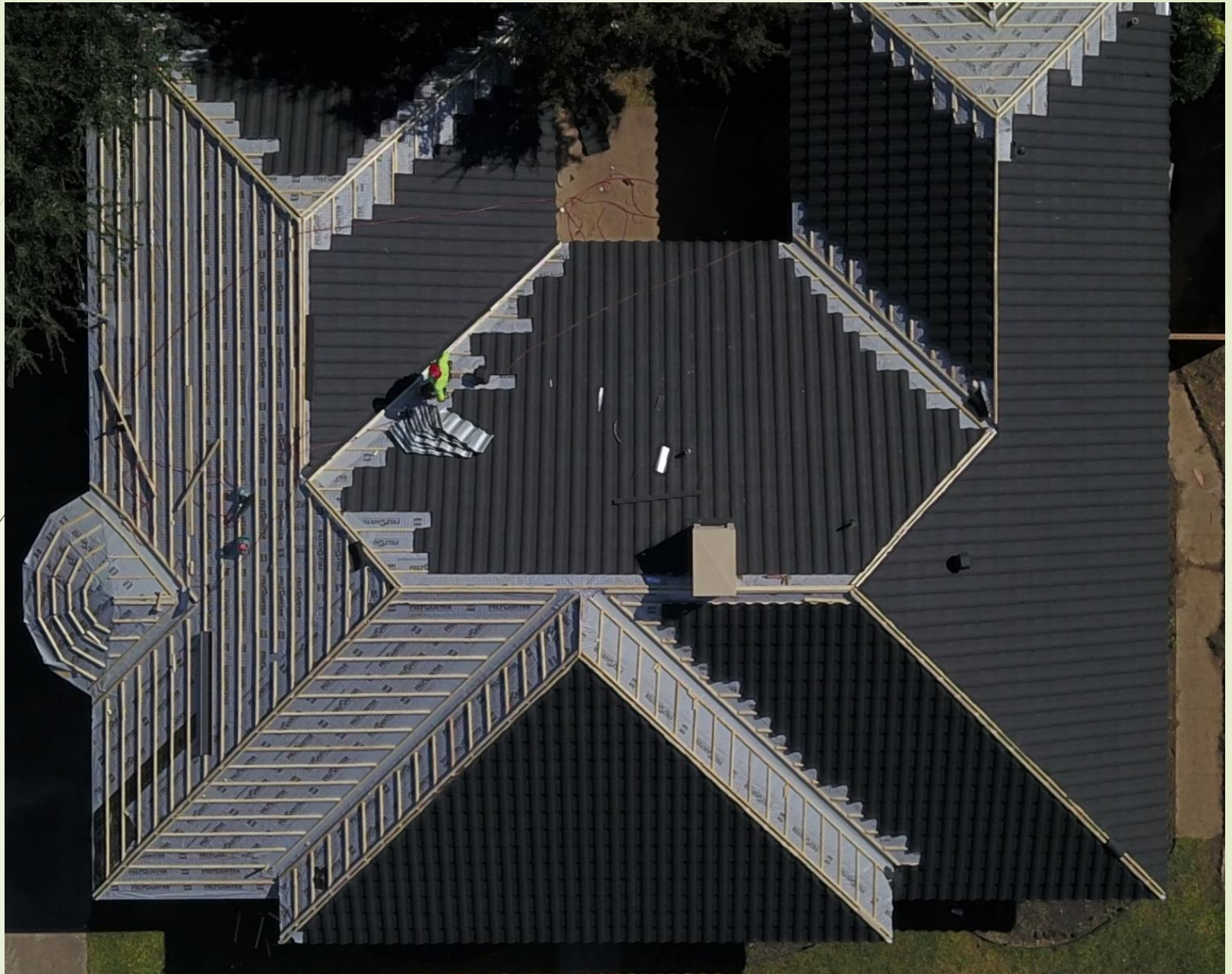
Overhead view of Cleo Tile installed on battens, engineered for fit and performance
